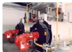
Measuring and control, DDC function
