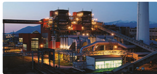
Control of central heating system – Martin Slovak Republic
