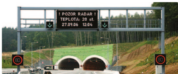
Highway tunnel Valik control Czech Republic
