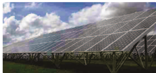
35 MWp photovoltaic power plant control – Veprek Czech Republic
