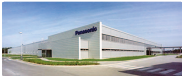
Heat and air-conditioning control system – Panasonic Czech Republic
