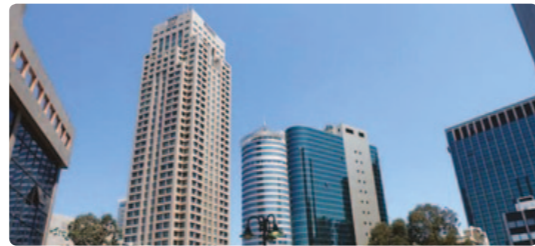
Air conditioning control system – administrative center Ramat Gan – Tel Aviv, Israel
